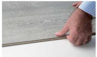
Hit gently with a soft-face mallet on both end joints and start by tapping the outside edge and moving inward to engage the plank.
